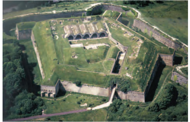
Aerial view of the Drop Redoubt showing accommodation casemates, ramparts and caponiers
